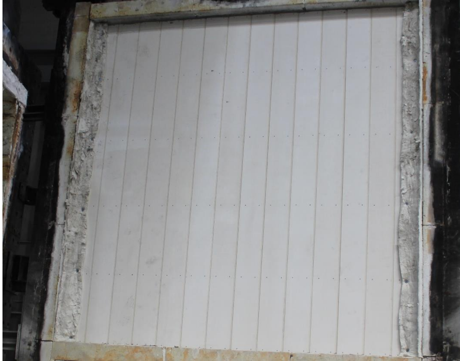
Figure 12 – Exposed face prior to test commencement
