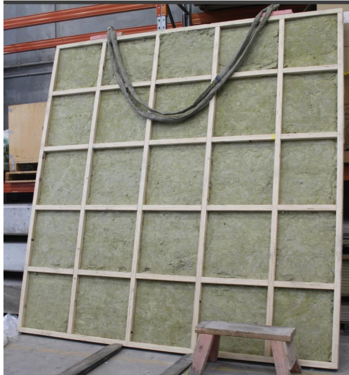
Figure 8 – Framing and insulation installed.
