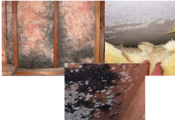
Figure 2 Three examples of interstitial condensation
